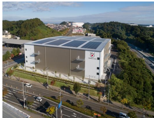
Example of the construction of a logistics facility
