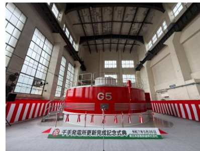
Equipment renewal work at JR East Shinano-gawa Power Station (Senju Power Station)
