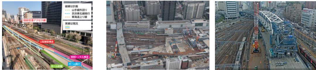
Haneda Airport Access Line
